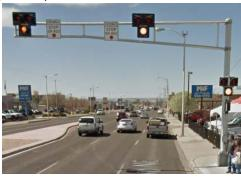
d) **Standard Traffic Signal.** An intersection must meet one of several criteria in the Manual on Uniform Traffic Control Devices (MUTCD) in order for a signal to be installed. For school crossings, at least 20 students must use the crossing, and it cannot be within 300 feet of another signal. The MUTCD also requires that other measures be considered prior to installation of a signal.
